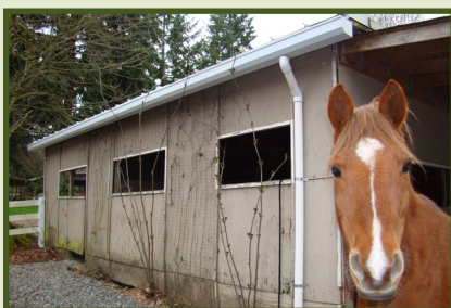
Roof Runoff Structure
